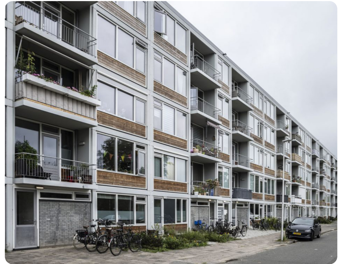
Fig. 11 Residential block of housing corporation Portaal in Utrecht (Photo by Duic)
