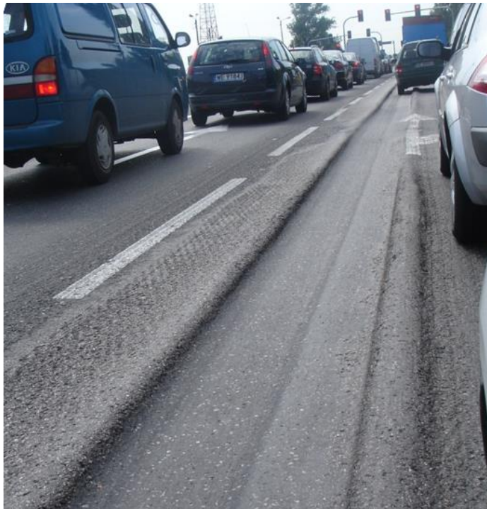
Figure 2-5: An example of rutting (Rotated and cropped, user Burda, CC BY-SA 3.0, via Wikimedia Commons)
