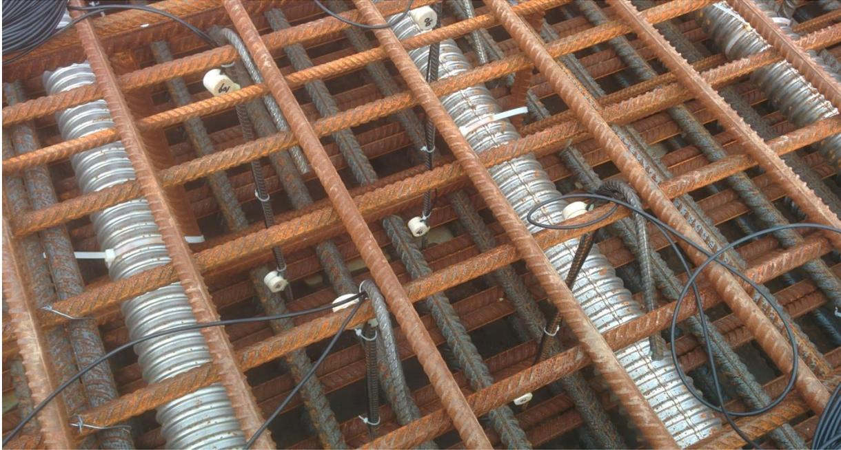
**Figure 9: Cane-shaped reinforcement bars with Smart Aggregate placed within the reinforcement cage of the bridge deck and glued in fixed position before concrete cast**
