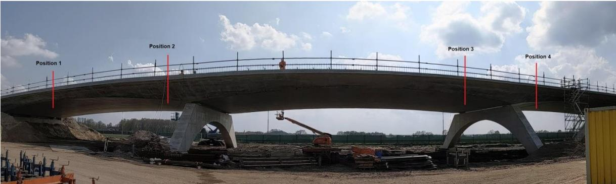
Figure 7: Panoramic side view of the concrete bridge from the construction site and the four illustrated positions of the four sensor groups within the measured spans of the concrete bridge
