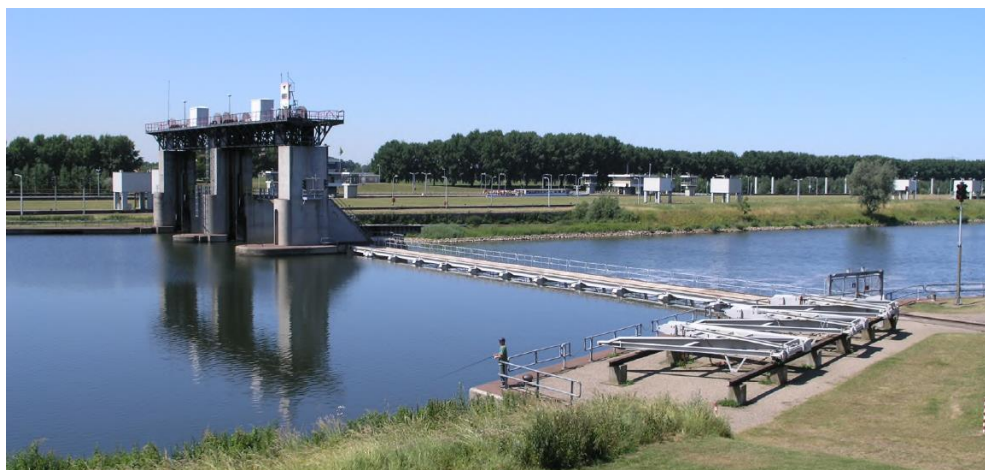
Figuur 14 - Stuw Belfeld (IV-Infra,2010)
