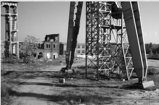
Figure 3. "C-mine" Cultural Square, Genk, Belgium
