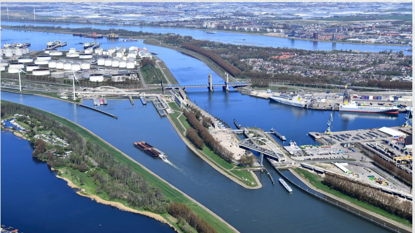
Figure 6. Aerial photo Theemwegtracé - Botlek
