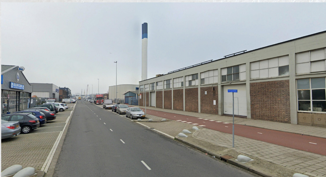
Figure 103. Transformation of a port area (Wastescape), polluted in Oud Charlois into a more green and ecological one. Before.
