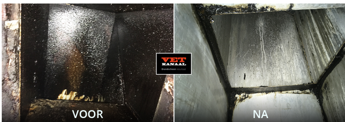
Figure 1-1: A comparison of an extraction channel before and after it is cleaned [1]
