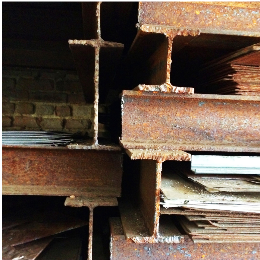
Expose metal cut
