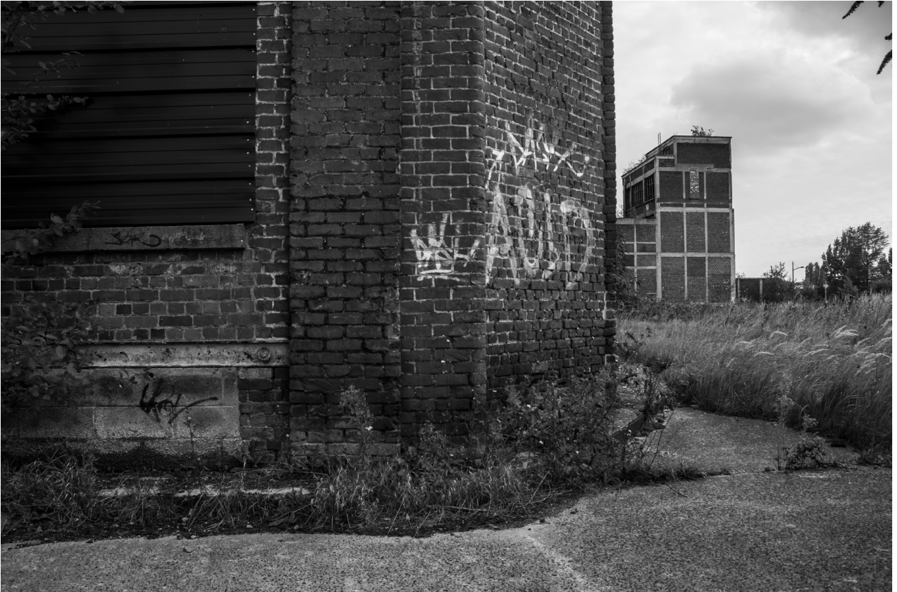
Ruins of the former textile factory Desurmont et Fils by author. 2017. Tourcoing, France
