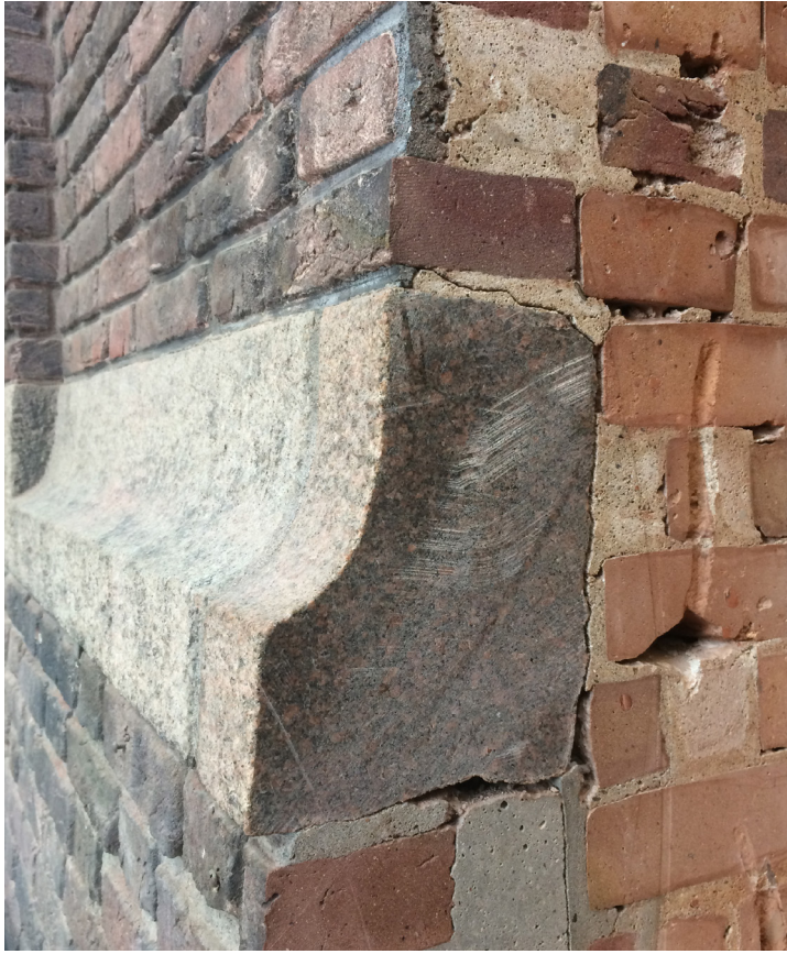
Expose brick cut
