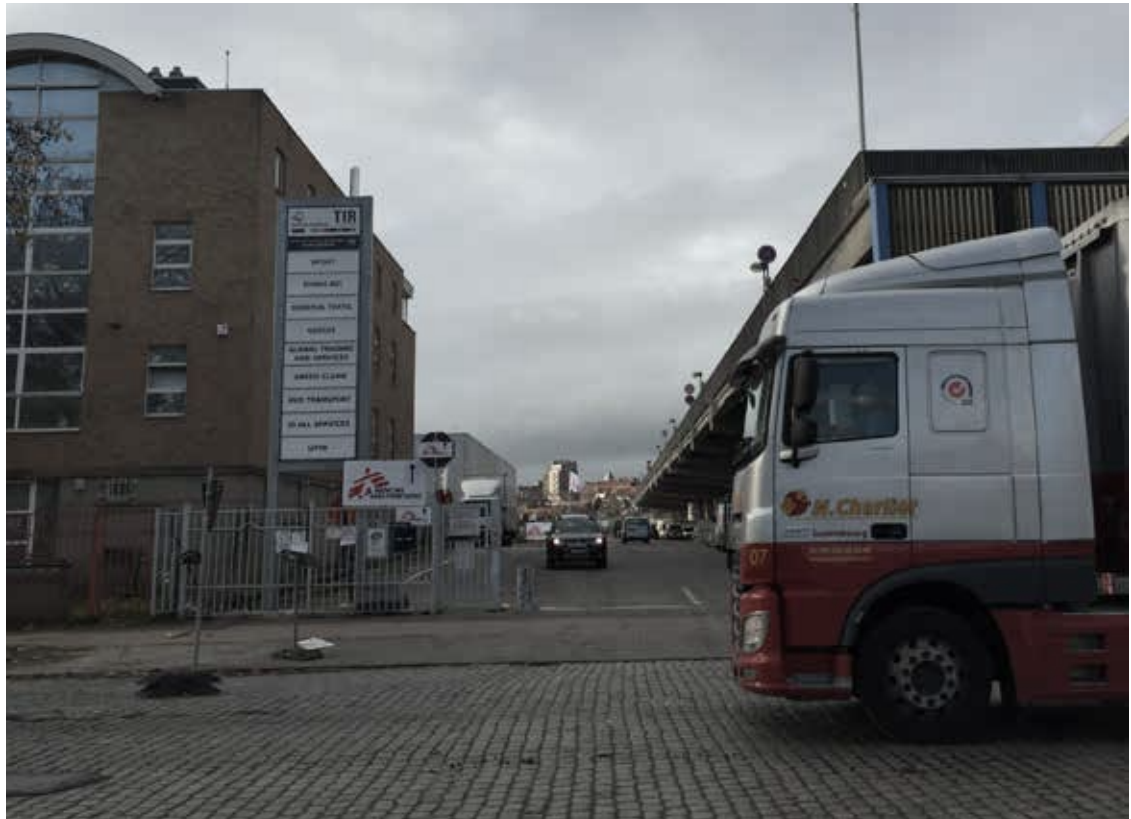
The TIR Site, an important logistics hub for the city which will soon be combined with circular economy initiatives © Adrian Hill
