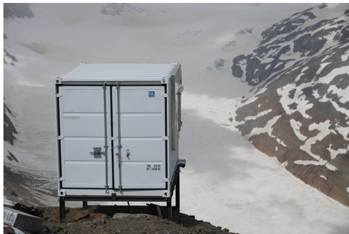
Figure 3.2: Container at the Im Hinteren Eis accommodating the scanning instrument and supporting facilities. This photograph is taken during a visit to the scanning system on 3 June 2022.
