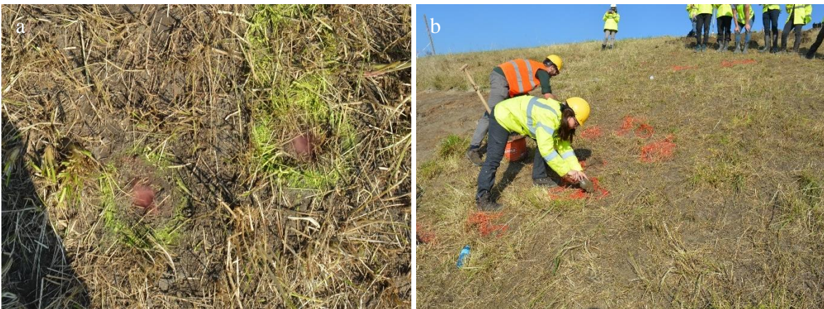
Figure 8: (a) Smoke emerges from two burrow openings. (b) The burrows that were emitting smoke were closed off with wet clay.
