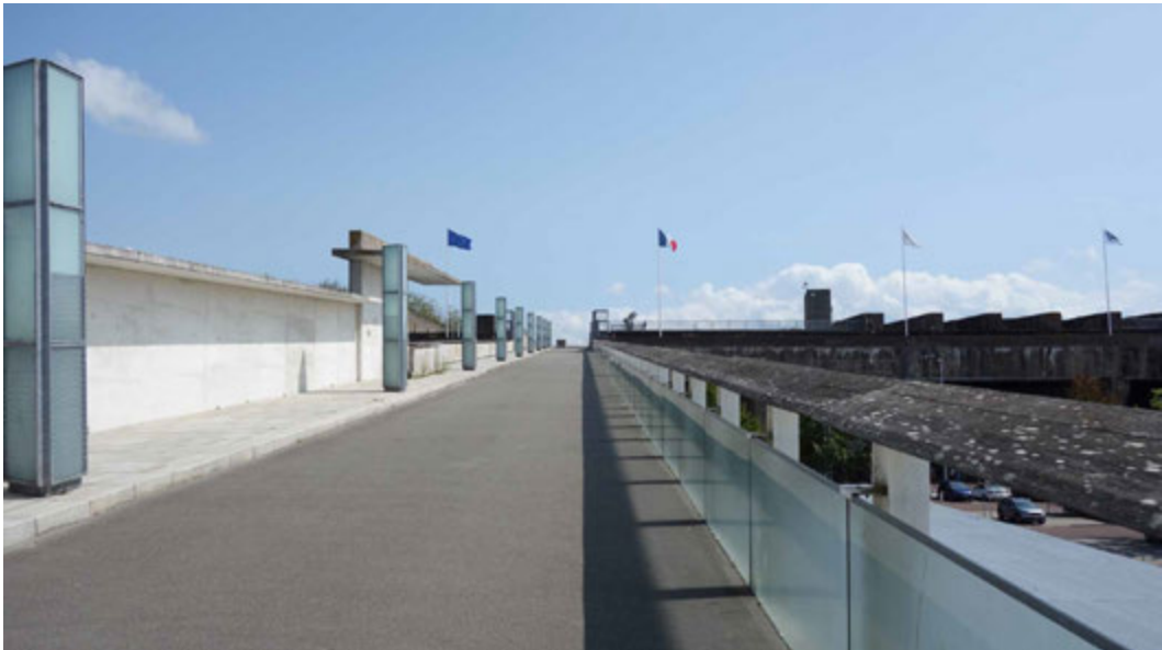
FIG. 5.22 The ramp to the roof
