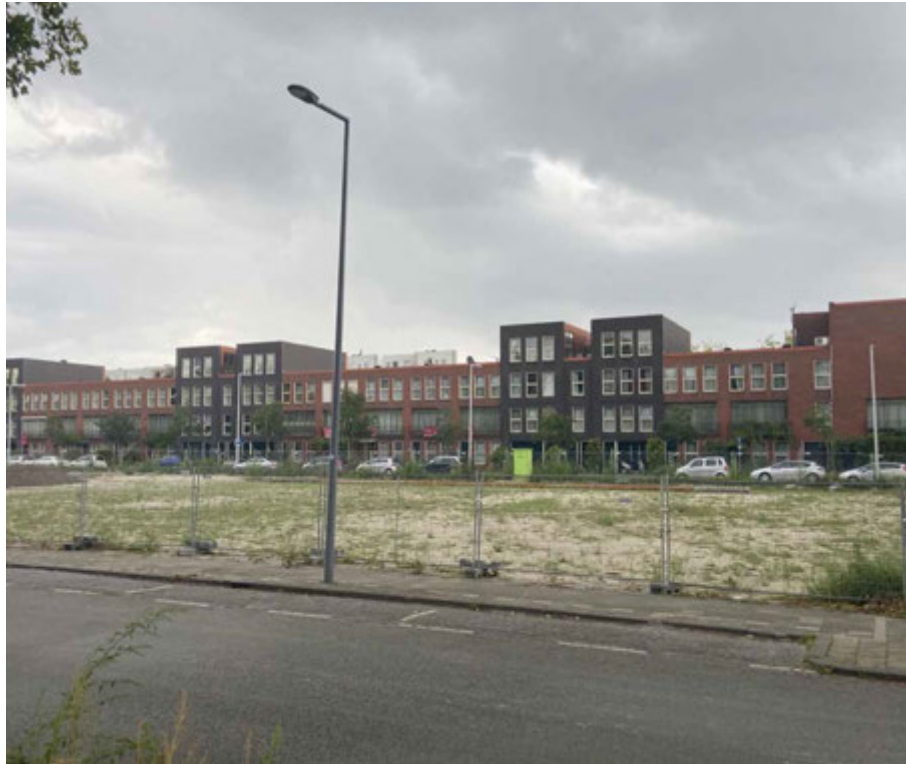
FIG. 1.2 Leftover space as spatial-temporal interstice, Mathenesse Vierhavensstraat, Rotterdam After the previous building blocks were pulled down in 2003, only the north area of the site was built on with new residential apartments, leaving a small piece of empty ground unoccupied for over 15 years. In 2020, the new housing development began, marking the end point of this urban interstice.
