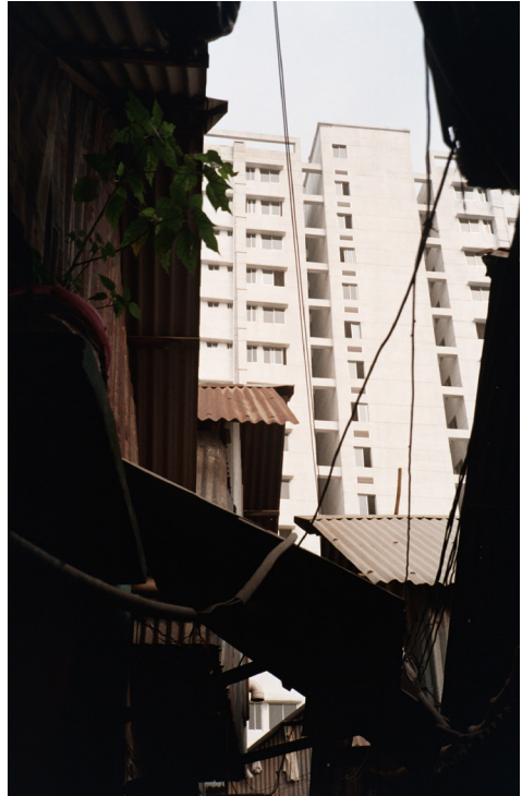
Fig.x: Government-Provided Housing building in contrast with the settlement, Dhaka, Bangladesh (Author, October 2023)
