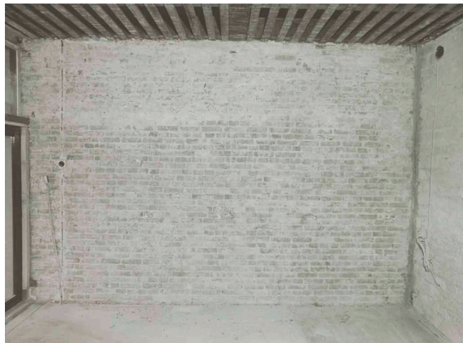
FIG. 3.6 Bare brick wall and stripped ceiling
