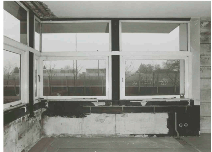
FIG. 3.4 The corner window during the restoration, with a view of the viaduct and the houses on Erasmuslaan
