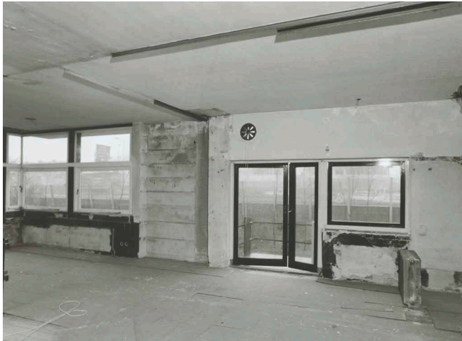
FIG. 3.3 The partially dismantled upper floor
