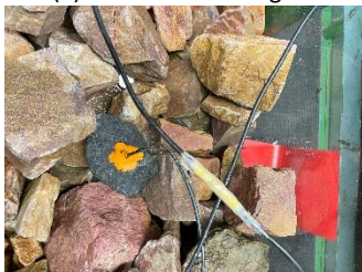
(g) Installing cameras in filter layer
