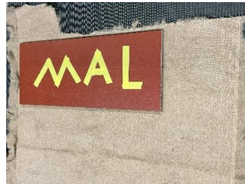
(b) Cutting geotextile to size
