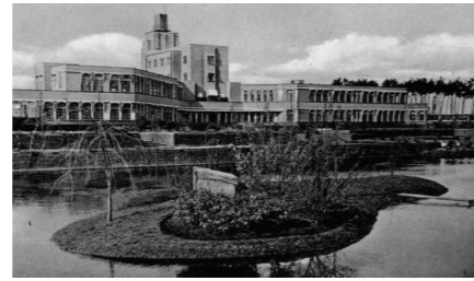
Sanatorium Noorder-Sanatorium, Drennoord
