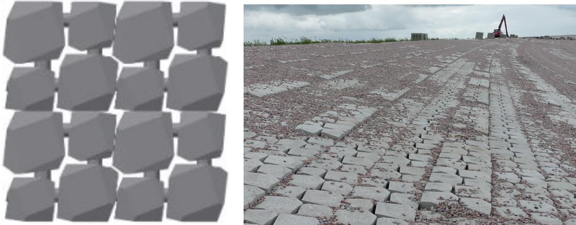
Figure 3.6: Set of Quattroblocks (left) and the placement on the upper slope of dike section 17 (right), Holcim Coastal B.V.
