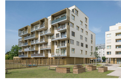
Zwei+plus Intergenerational Housing
