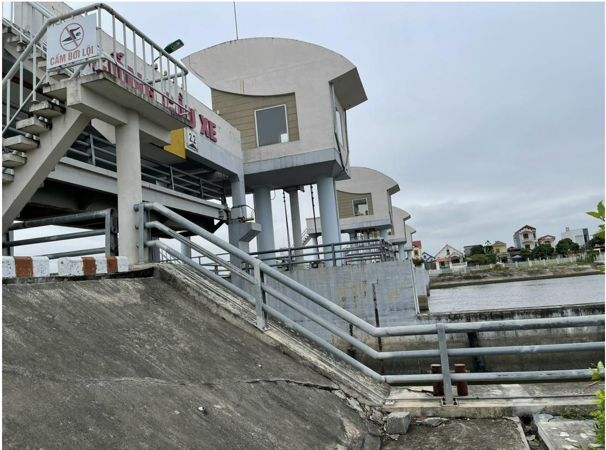
Figure C.2: Sluice leaks due to bad concrete conditions (Cong Cau Xe Moi)
