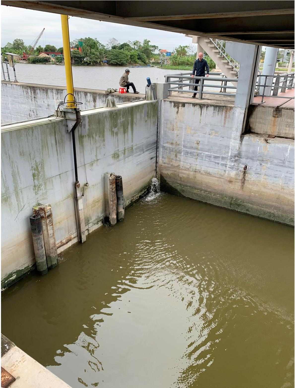
Figure C.3: Sluice leaks due to bad rubber conditions (Cong Cau Xe Moi)
