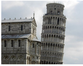
(a) Tower of Pisa in Italy with a tilt angle of 4^\circ (Lintula, 2006).
