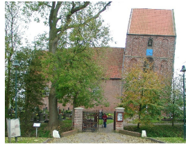
(b) Tower of Suurhusen in Germany with a tilt angle of 5.2^\circ (Heymann, 2004).
