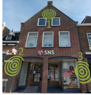
Figure 4.20.: Location of the three points on the facade mentioned in Table 4.4.
