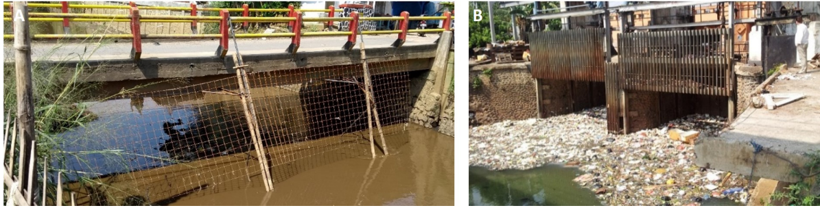
Figure 3.4: (A) Temporary trash rack construction installed by the military in the Cikapundung River in Bandung compared to commonly used trash racks, (B) such as the Mangarai Gate in Jakarta (Pagano, 2011)
