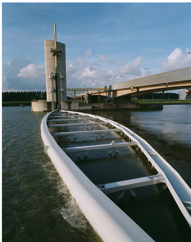
Fig. 5. Hartel Barrier. (Image © Rijkswaterstaat, used with permission.)
