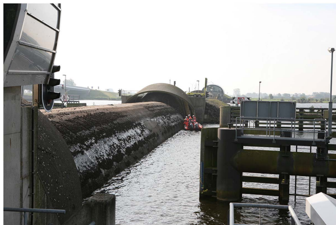
Fig. 6. Ramspol Barrier. (Image © Rijkswaterstaat, used with permission.)
