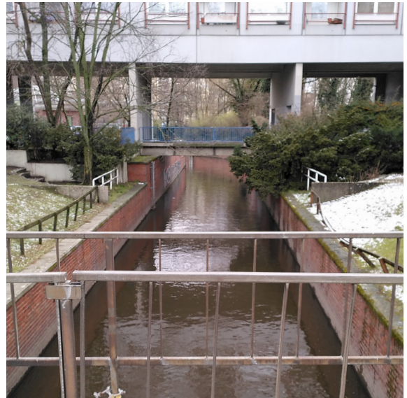
Figure 4.3d. Building above the water
