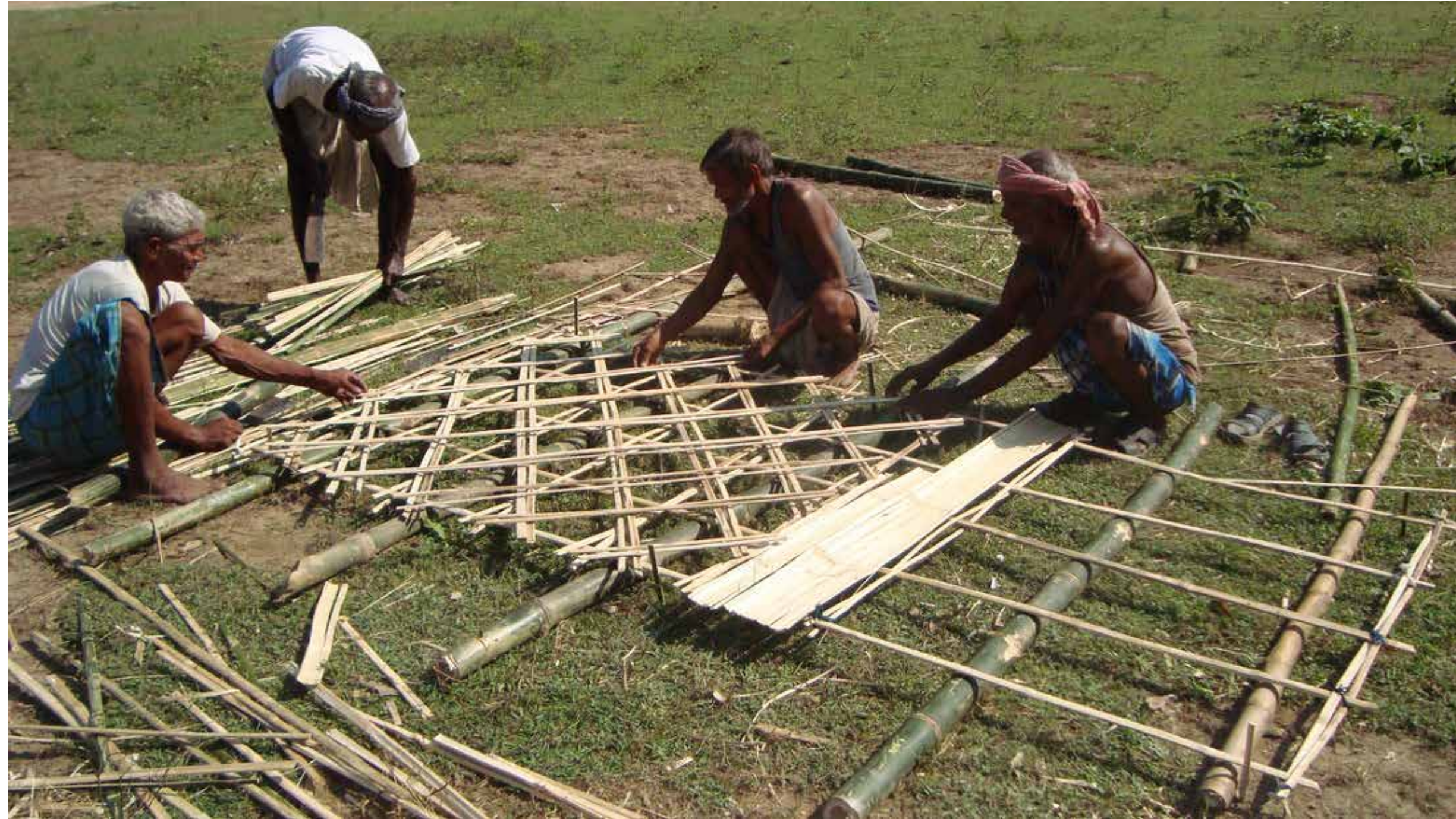
Local Craftmen can contribute by weaving the panels for the second facade.
