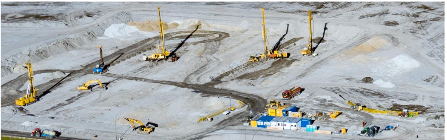
Figure 6 - A TSF of a copper mine located in Żelazny Most in Poland that has been in operation since 1977. This is the largest TSF in the European Union, and one of the largest TSFs worldwide. The immense size of this TSF is illustrated by the zoomed in part of the photo that reveals tractors, trucks, and other large size construction equipment on top of the dam.
