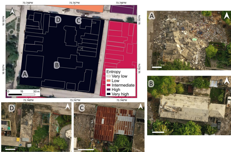
Fig. 6 Close up to a city block showing a very high level of average entropy texture. The close up corresponds to the area 2 highlighted in Fig. 4. Imagery data A, B, C, and D correspond to buildings visually inspected in a 2-cm-resolution drone orthophoto acquired on 18 August 2021. Building footprints within each block are outlined in grey
