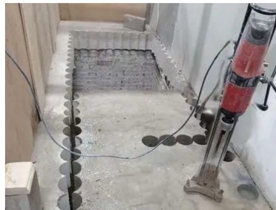
(b) Example of stitch drilling in practice
