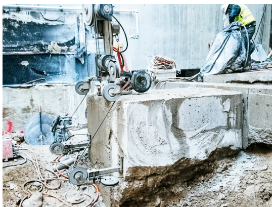
(a) Example of a wire saw being used in practice
