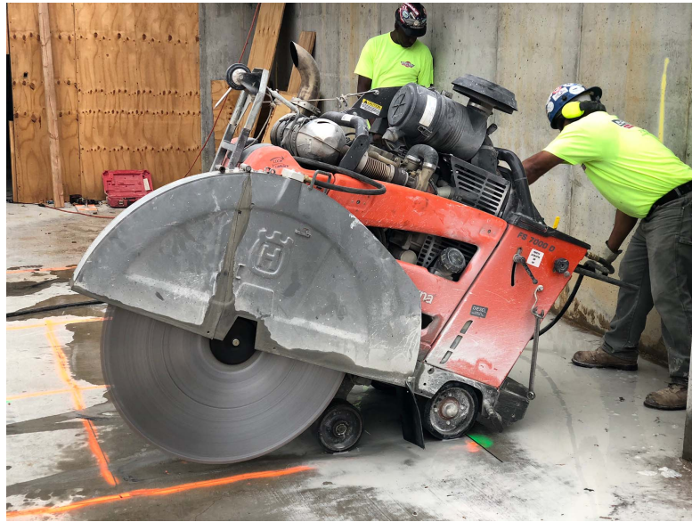
Figure 2.24: Example of a slab saw being used in practice
