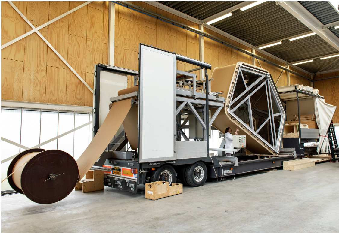
Construction process of the paper-based Wikkelhouse - Fiction Factory (2012)
