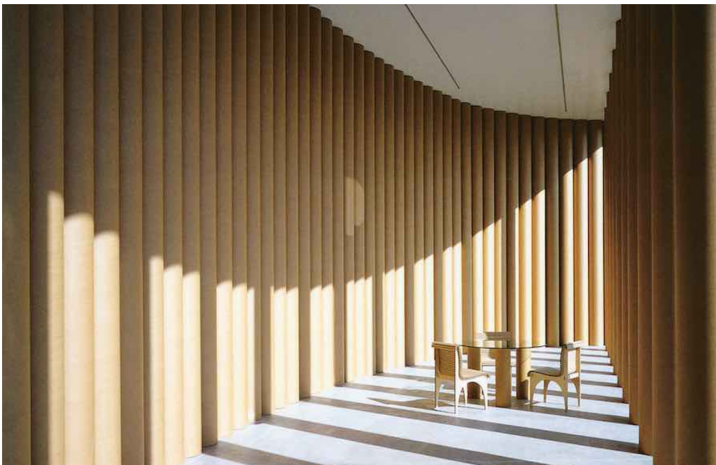
Paper tube roof and wall constructions: 1. Disaster relief center, S. Ban (2013). 2. Ring Pass Delft, Octatube (2010). 3. MDS Gallery, S. Ban (1994)
