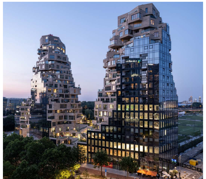
Picture 1 | The Valley by MVRDV Van Duivenbode, S. (2022, 20 September). Valley Towers / MVRDV . Found on https://www.archdaily.com/989217/valley-towers-mvrdv
