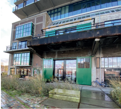
Entrance to dwelling on ground floor
