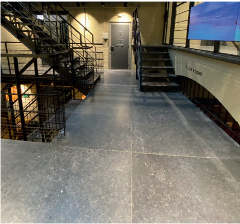
Large stone tiling finish in circulation space of library
