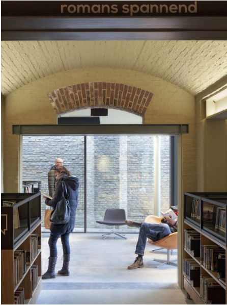
New opening is existing wall
