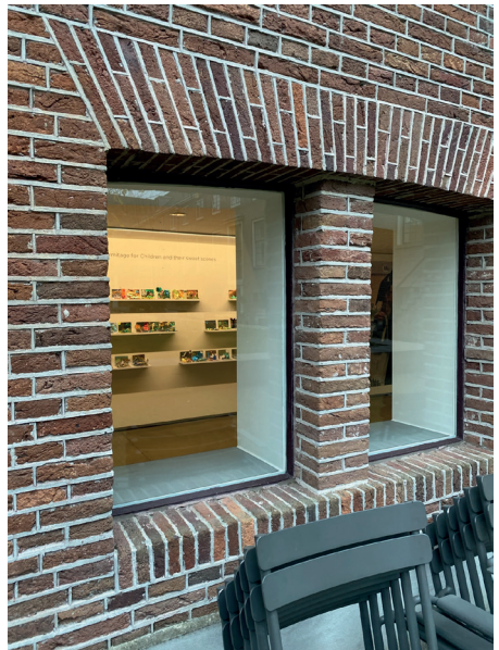
Windows creating views to interior
