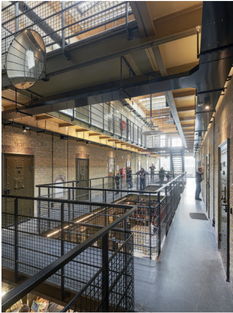
Existing void in shops (block H)
