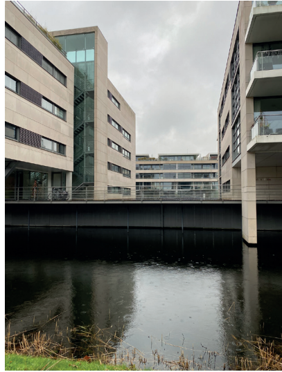
Staircase and void with curtain wall
