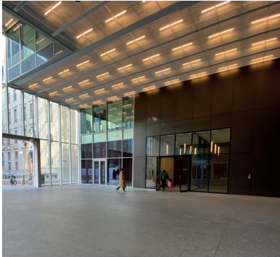
Entrance passage to dwellings
