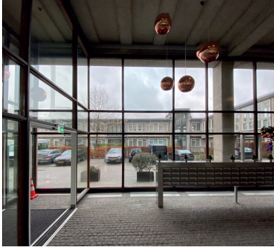
Double height curtain wall
