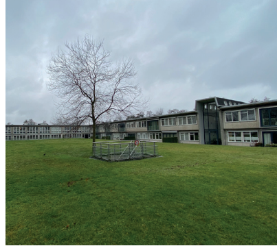
2. Former laboratory halls
