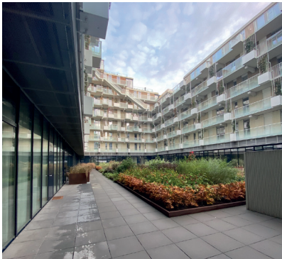
3. Courtyard elevated above warehouse
