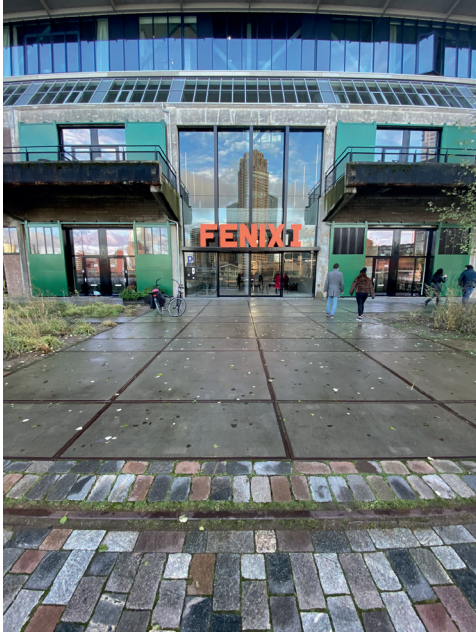
Entrance of passage waterside
