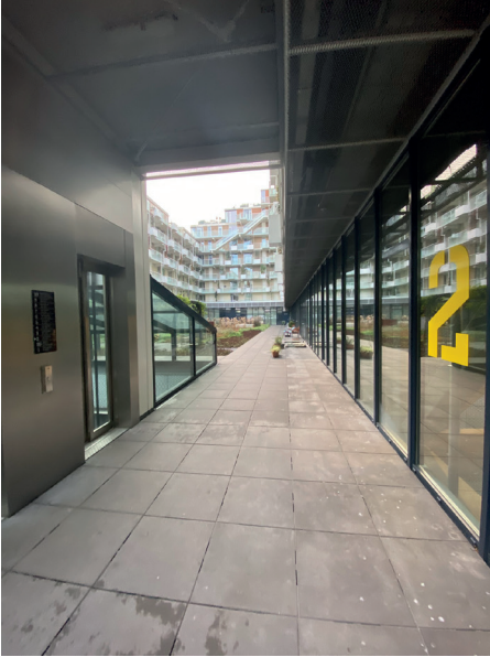
Courtyard of dwellings on third floor
