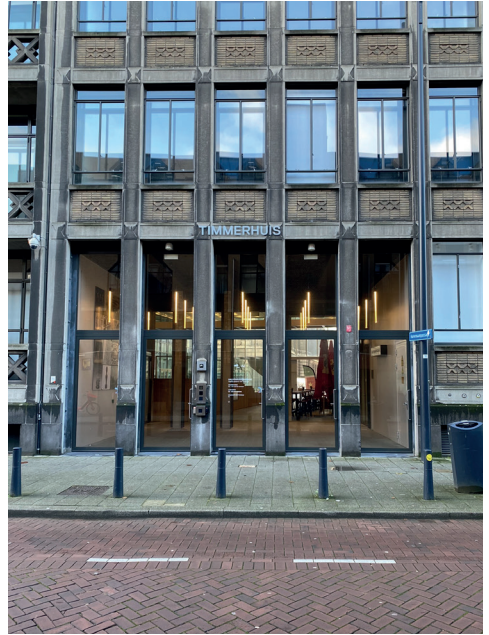
Entrance passage existing volume
