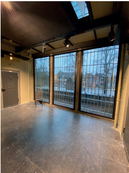
Replacement of existing windows
