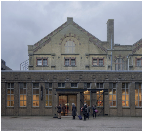
3. Entrances in former forge
