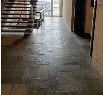
Stone tile finish in hallway main building
