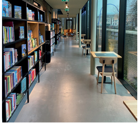
Polished concrete floor finish in added part of library
