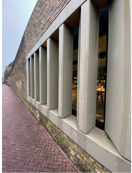
Openings in wall creates small views to inside
