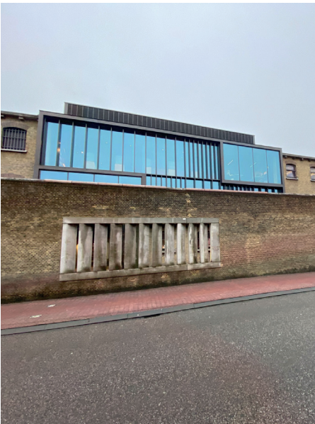
Intervention in facade of library
