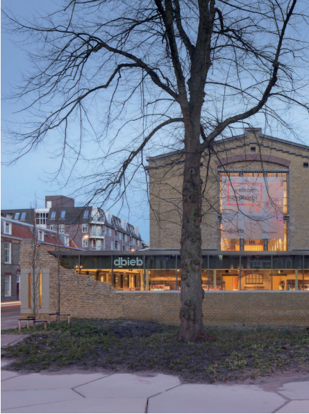
Visual connection as result of collapsed wall
