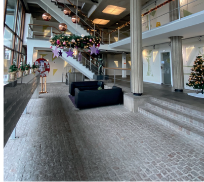
Stone floor finish in entrance area
