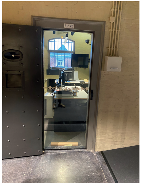
New glass doors and windows in cell doors
