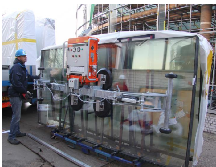
Figure 23: On site bending using a robotic vacuum machine (Bijster, Noteboom, & Eekhout, 2016)
