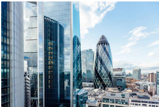
Figure 1: Fully glazed facades, London (Spatari, 2021)
