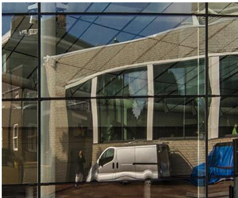
Figure 33: Visual distortions due to anticlastic bending (Octatube, 2015)
