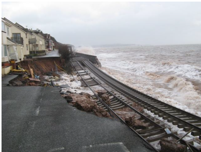
FIGURE 5 (a) Retaining wall collapse at Kupjak Tunnel, Croatia (Gavin, 2016). (b) Sea wall failure at Dawlish, Devon, UK; image © Network Rail
