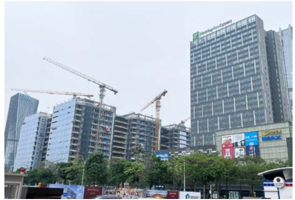
The town centre under construction
