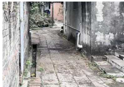
[Fig.6.35] Domestic sewage pipes laid under the street
