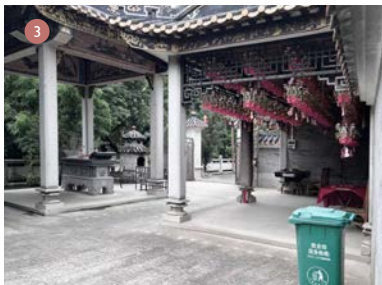
[Fig.6.21] Cultural building used as leisure place
