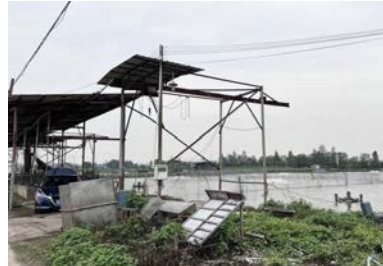
[Fig.6.31] Cable setting in the fish pond
