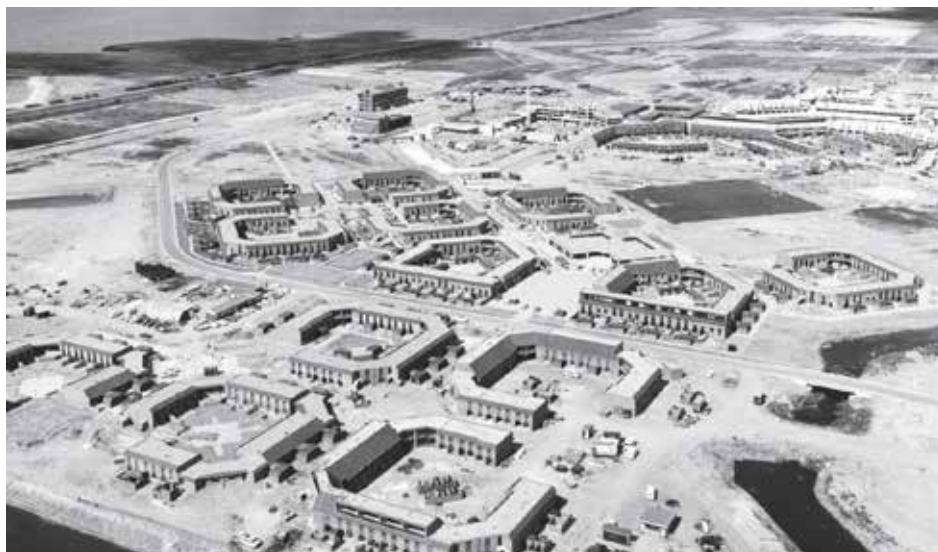
Figure 2. The construction of De Werven in 1976. A bloemkoolwijk in the groei kern of Almere. Source: Stadsarchief Almere
