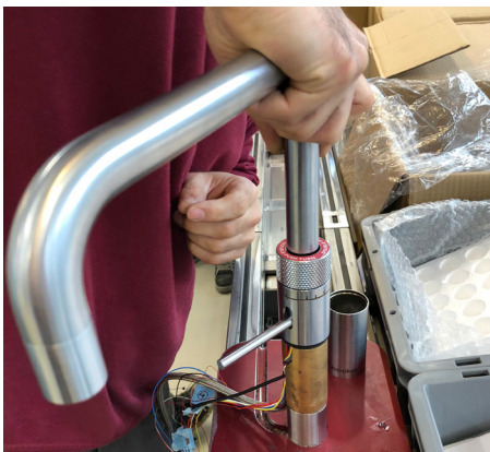
Step 7: attaching the outlet on the tap.
