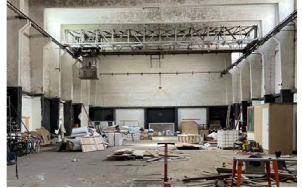
Concrete portals and trusses
