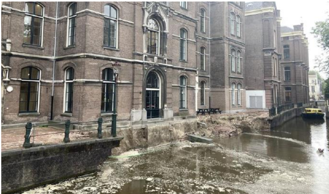
Figure 3.1: the Grimburgwal after collapse from the research of Korff et al. (2021).
