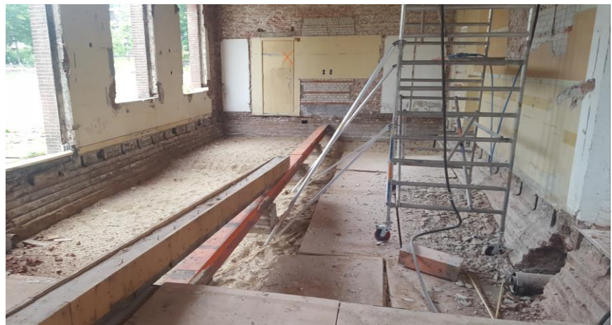
Figure 5.6: Before situation of the foundation (Res & Smit BV, 2016)
