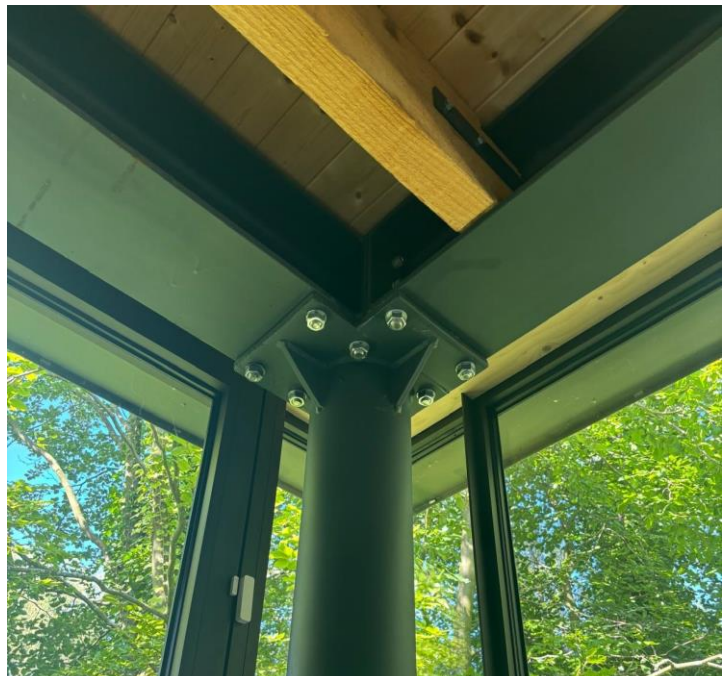
Figure 5.16: Detail of dismantlable element (own photo, 2024)
