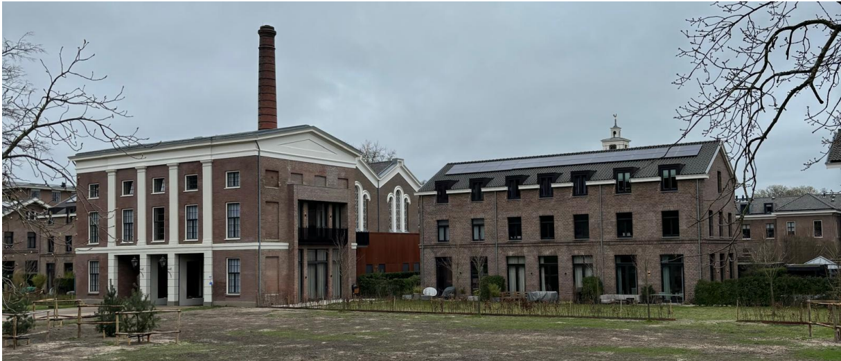
Figure 5.2: Newly built part (right) and existing part (left) (own photo, 2024)
