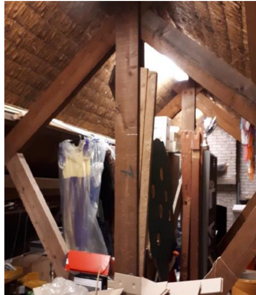
Figure 6.10: Old situation of the attic used as storage space (Bouwer, 2017)
