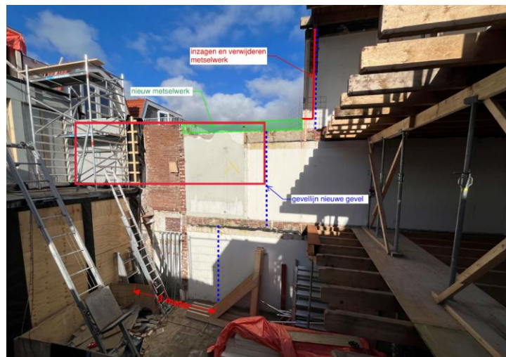
Figure 5.37: Situation during construction process (Res & Smit BV, 2021)
