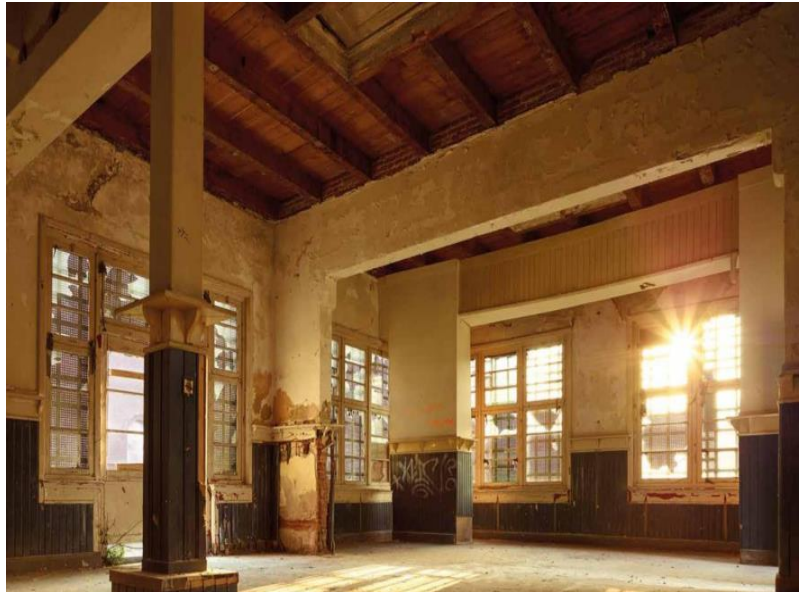
Figure 5.7: High ceilings in the before situation (Res & Smit BV, 2016)
