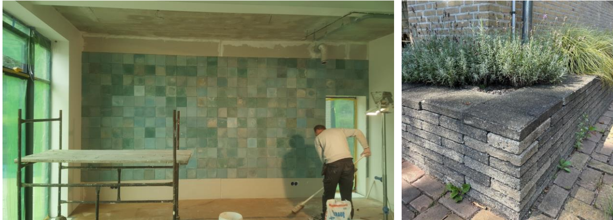
Figure 5.24: Second-hand tiles for interior (left) and exterior (right) (Res & Smit BV, 2018)
