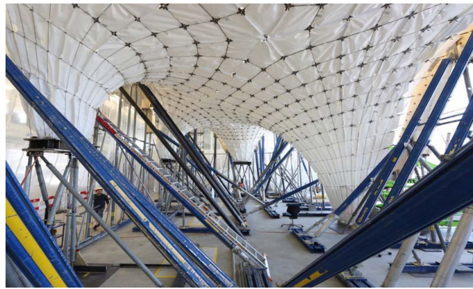
Figure 7. Construction of the NEST HiLo prototype. (Source: Block Research Group)
