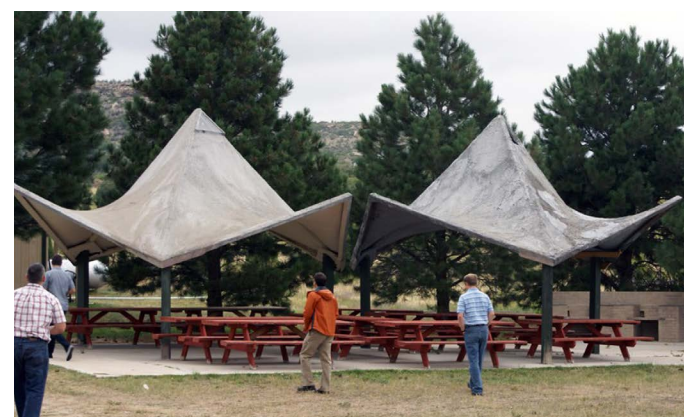
Figure 34. Diagram from a 1975 patent for flexible formwork using a rigid frame (Kersavage, 1975), (B) Construction of a hypar roof shell using textiles stretched over a rigid frame (Source: TSC Global), (C) Completed flexibly-formed hypar roof shells by George Nez (Source: TSC Global)
