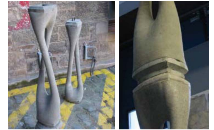
Figure 39. Flexibly formed columns where connections were strategically formed with rigid plastic molds to facilitate easy aggregation (Pedreschi, 2011)
