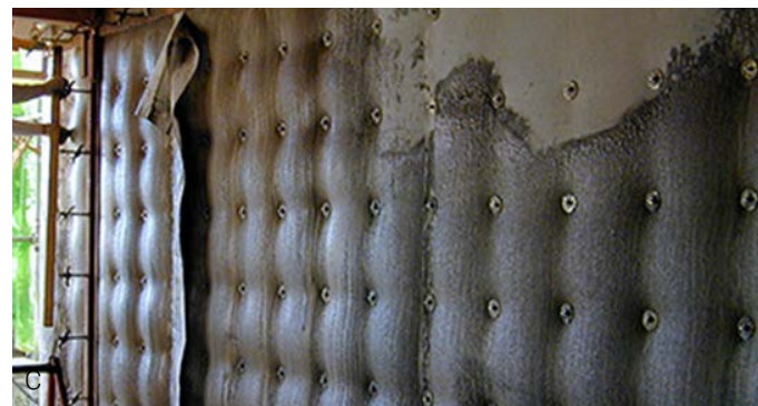
Figure 26. Flexibly formed walls by Kenzo Unno. (A) Frame Method, (B) Quilt-Point Method, (C) Partially filled quilt-point mold (Source (all): Kenzo Unno)
