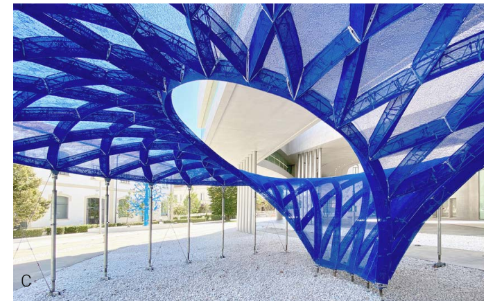
Figure 3. Various CNC knit formwork prototypes. (A) Concrete shell bridge (Source: Block Research Group), (B) KnitCandela Pavilion (Source: Zaha Hadid Architects), (C) KnitNervi Pavilion (Source: Block Research Group)
