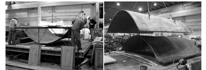
Figure 29. Hanging mold construction and flipped hardened element. (Source: Mark West / C.A.S.T.)
