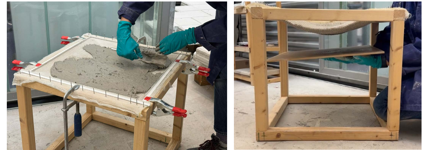
Figure 136. The manual nature of the casting process likely contributed to uneven deformations in the samples. (Left) Concrete paste is applied manually to the textile, (Right) The removal of the stabilizing plate often caused some areas of the textile to be released before others which might contribute to uneven deformation.
