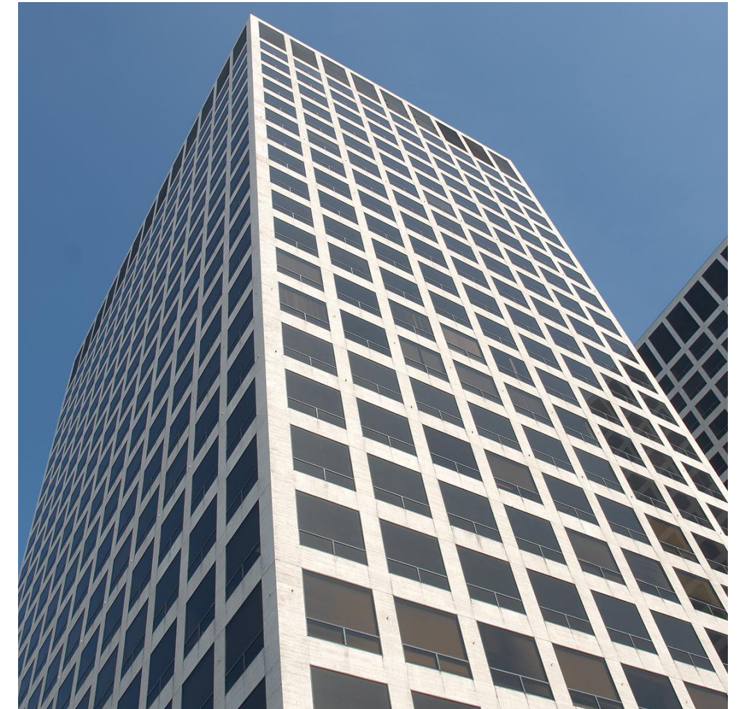
Figure 7.1: North-east view of the Rotterdam Science tower (ErasmusMC, 2015).
