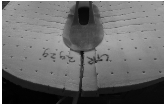
Figure 57 Cutting the opening in the topdeck layer.
