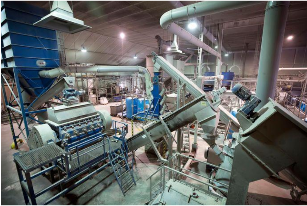
Figure 19: buildup of various shredders and separators at Coolrec in Dordrecht, NL (Verrijt, 2019)
