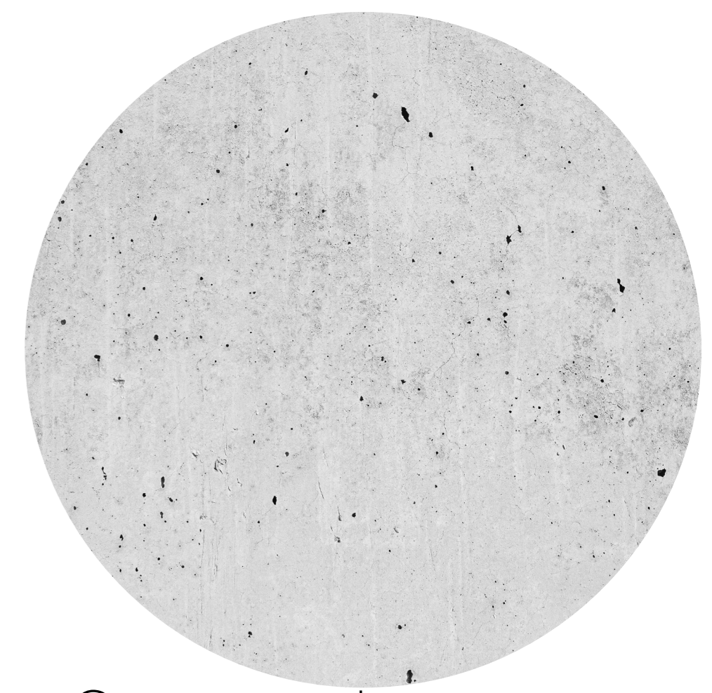
Concrete elevator core
