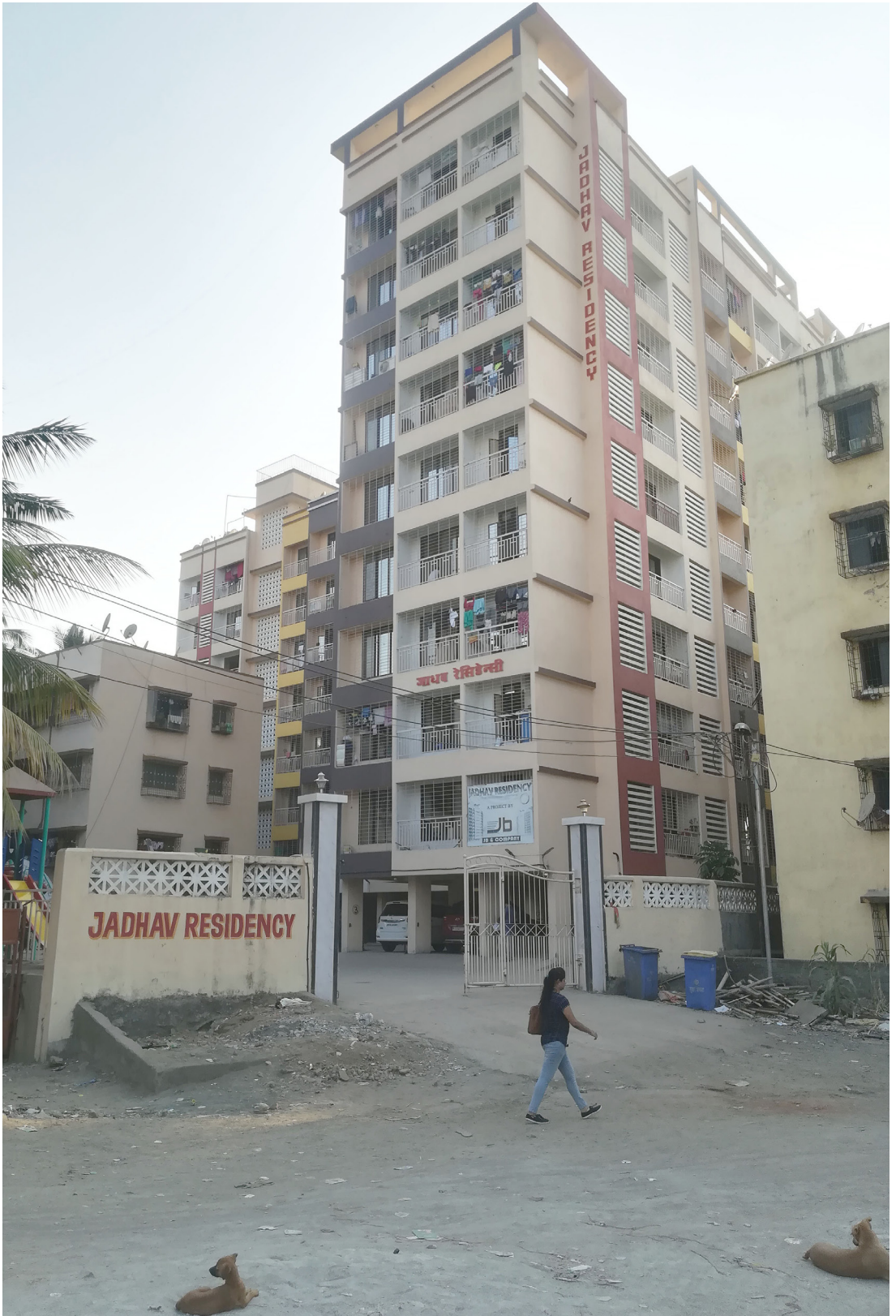
Rahmat Nagar. Newly built 10 storey apartment building
