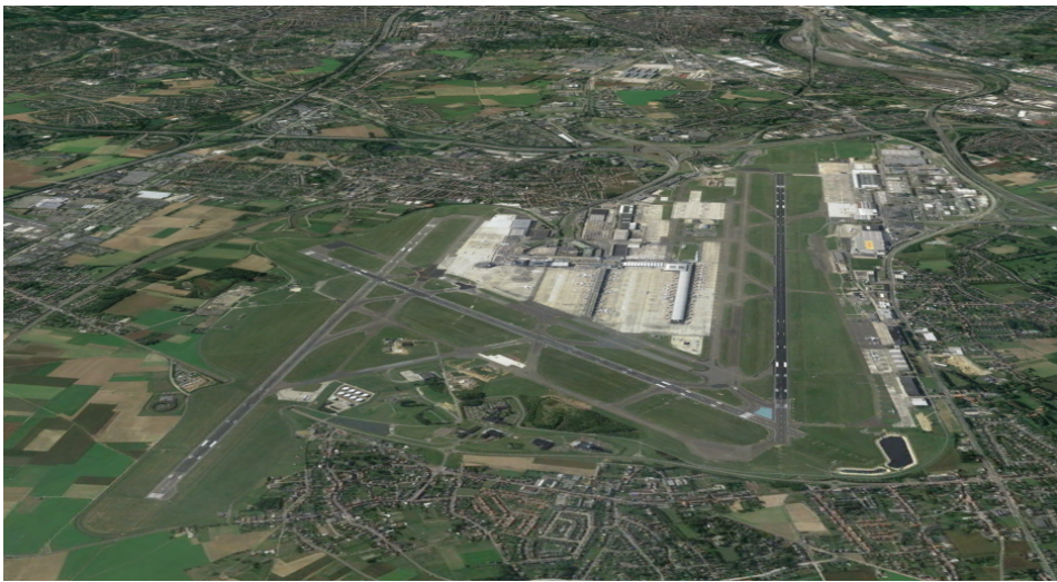
Figure 1.5: Overview of Brussels Airport Zaventem (source: Google Earth)
