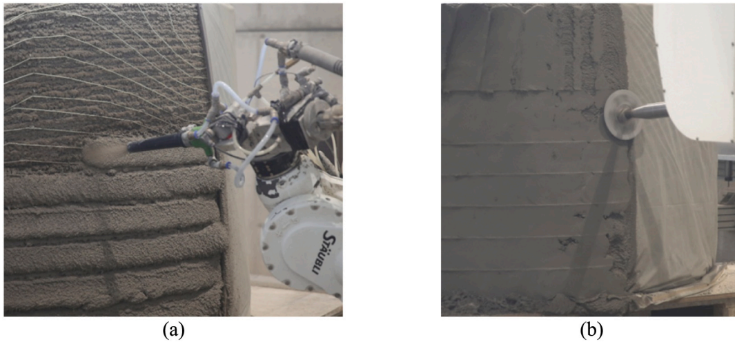
Fig. 24. Printing vertically onto a horizontally printed core: a) embedding the robotically fabricated fibre reinforcement; b) robotically trowelling the fresh concrete in a subsequent formative process, [101].
