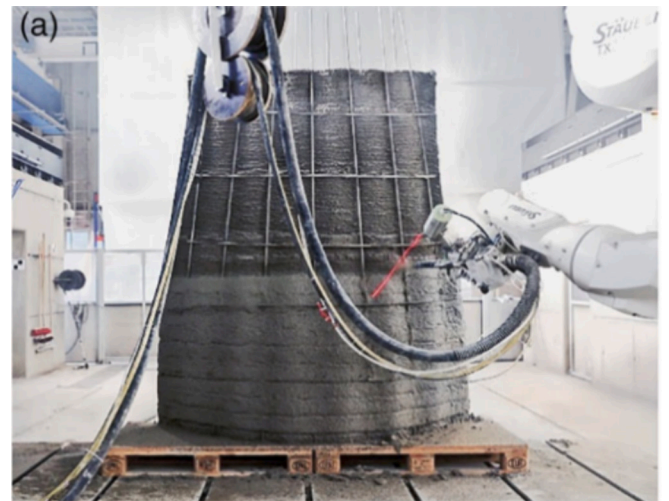
Fig. 7. Cover Layer Printing using Shotcrete 3D Printing (SC3DP, Technical University of Braunschweig, 2020) [27].
