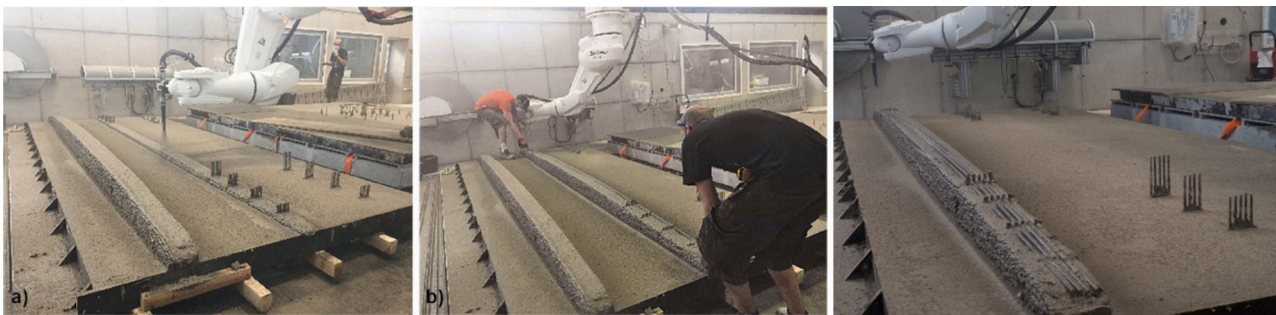
Fig. 10. (a) Add-on Printing of concrete ribs with varying cross-section heights (b) Application of the longitudinal reinforcement bars (c) Application of the concrete cover onto the reinforcement [29].
