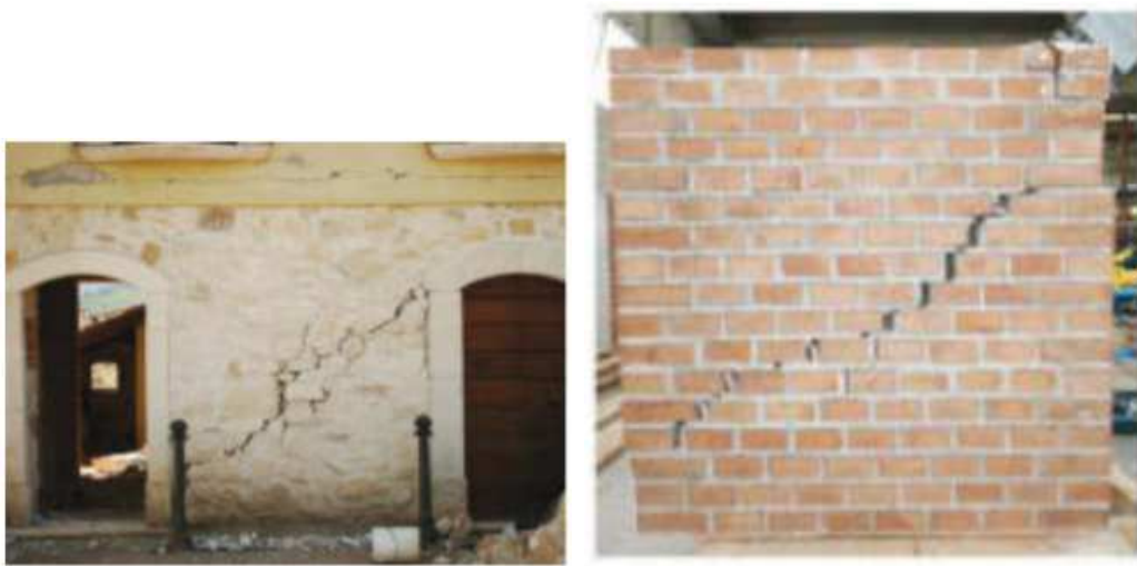
Figure 2.2: Detachment and sliding due to combined compression and shear [Angelillo et al., 2014]
