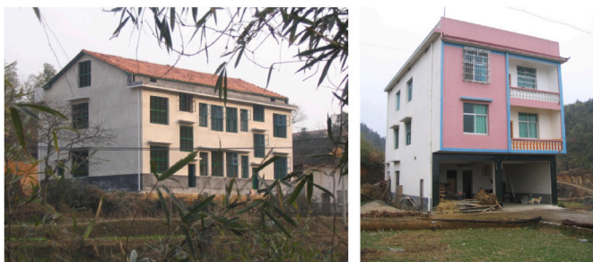
Fig. 1. Rural single-family buildings in northern Hunan Province.
