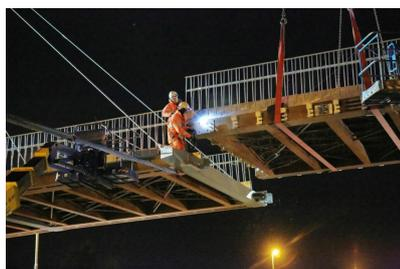
(a) Steel parts integrated in deck [38]
