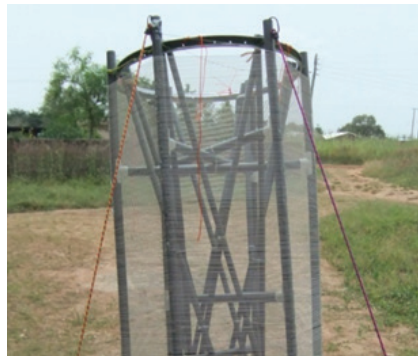
Figure 4.13: DTS cable set-up (Left) and DTS installed in the Lake (Right) at Binaba
