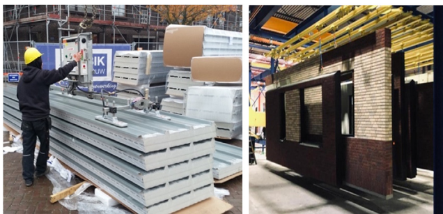
Figure 10.4 (A) Prefabricated roof panels used in the construction of the 12 zero-energy dwellings, in Vlaardingen, the Netherlands. (B) Completerc RC Panels ( Rc Panels, 2021 ) with weather finishing of brick tiles.
